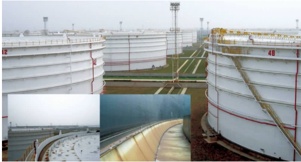
Fiber Bragg Grating temperature sensing fire alarm system in one of the oil reserve bases
